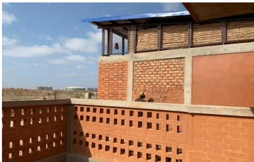
**Figure 19: Typha, a cane, can be used for insulation and in earth bricks**
