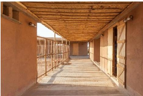
**Figure 17: Clay materials have excellent moisture absorption properties and increase thermal comfort in buildings.**
