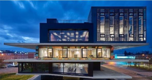
Figure 13: The Urban Mining and Recycling (UMAR) Experimental Unit is an experimental building mostly constructed with fully reusable, recyclable and compostable building materials. (Architects: Werner Sobek, Dirk E. Hebel & Felix Heisel, Photo: Zooey Braun)
