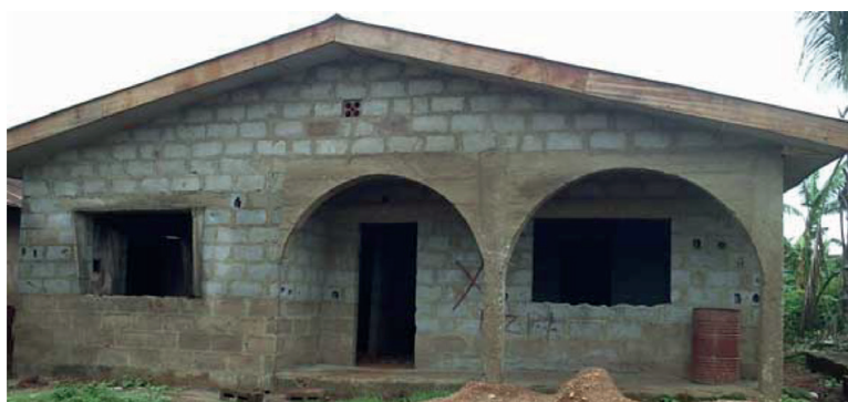
Figure 4. A typical building under construction using concrete hollow blocks.
