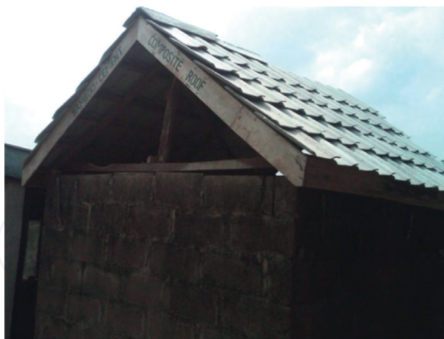
Figure 6. Fibre-reinforced composite roofing tiles installed on a gable-roofed building in Ibadan, Nigeria. Source: [23].
