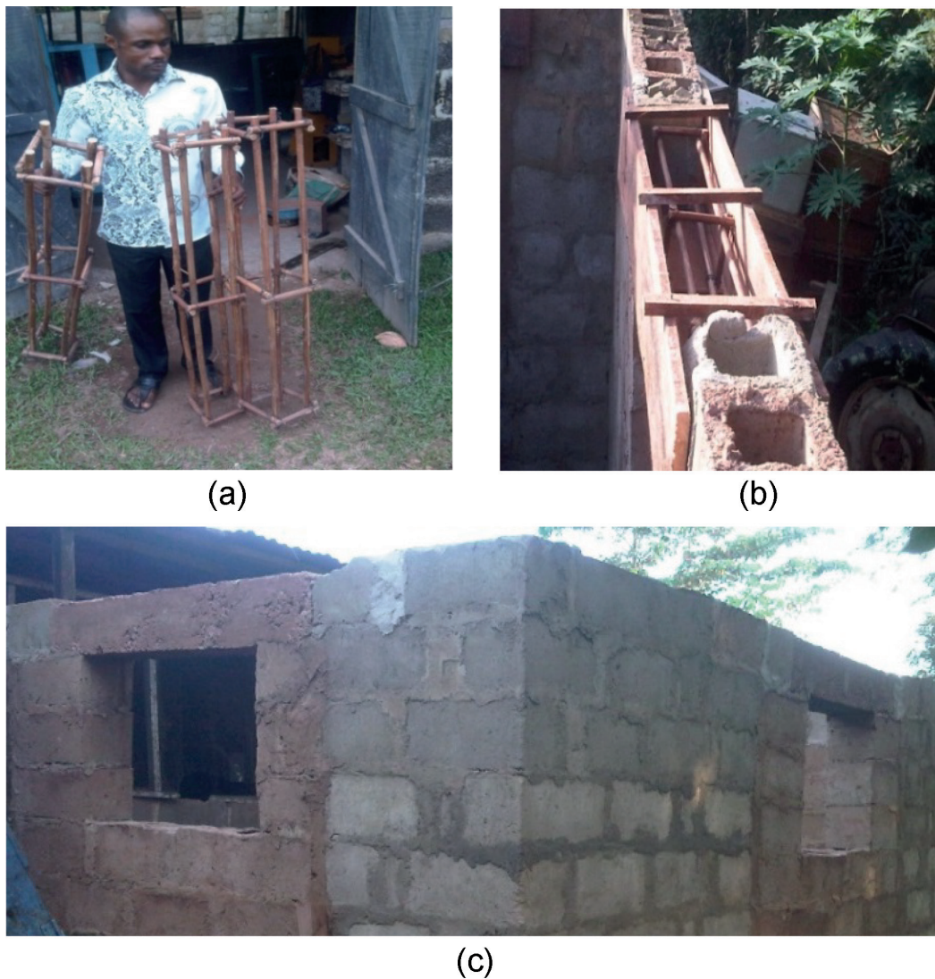
Figure 15. (a) Rattan cane reinforcement, (b) lintel beam casting in progress, (c) the cured concrete lintel beam after 28 days. Source: [23].
