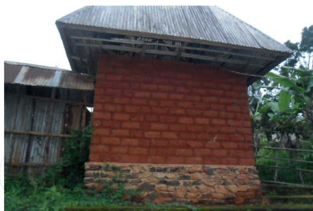
Figure 3. A typical building constructed using clay bricks.
