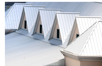
Cool Roof in Ottawa
