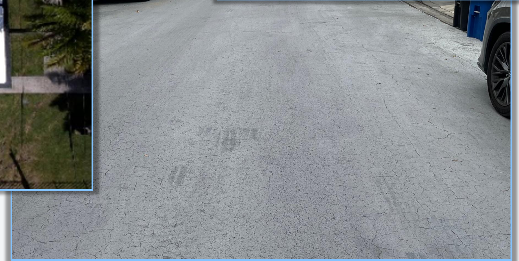
Cool Pavement Installation (Los Angeles) Photo credit: Cool Roof Rating Council
