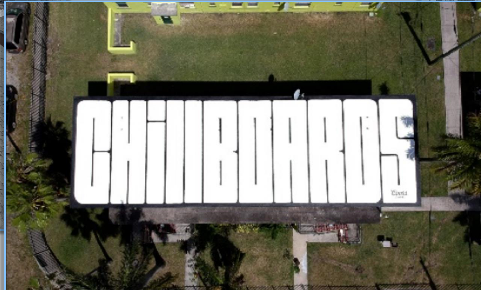
Cool Roof Installations (Miami) Photo Credit: Mule-Hide Products
