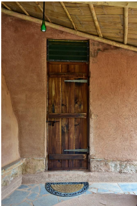
Left image: Fire bricks finished with thappi plaster for the walls.
