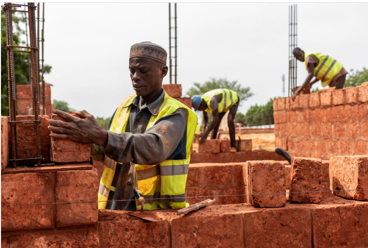
Construction using laterite stone blocks. Credit: Grant Smith
