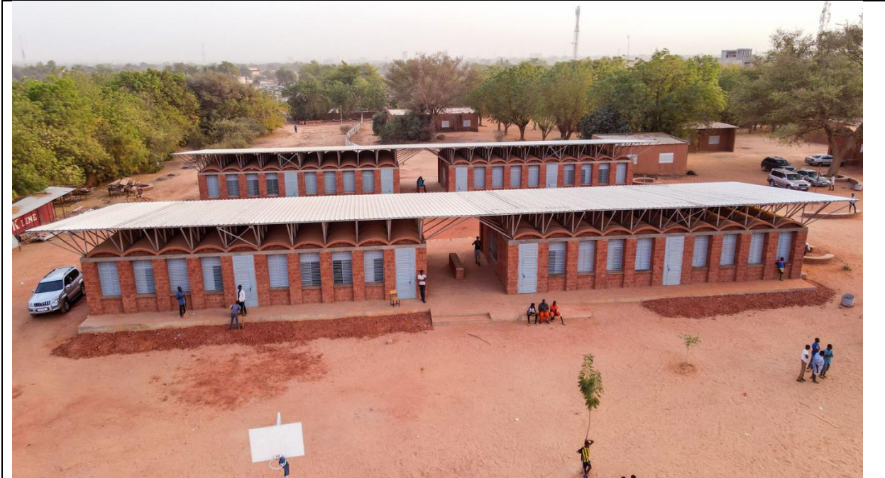
Aerial views of school buildings. Credit: Souleymane Ag Anara
