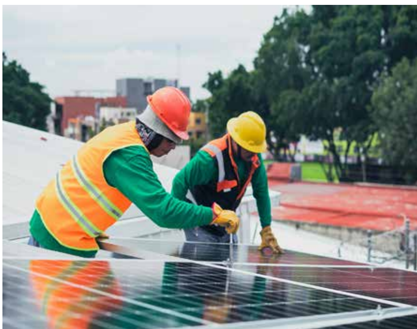
Figure 5-8: Solar Panel Installation
